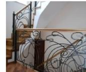
Fig. (5) Handrails were not fully extended non-continuous
