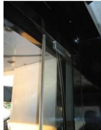
Picture 38 provided a break using rubber to reduce shock and friction resulting in cracking door leaf
