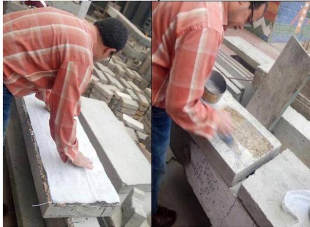
Fig(8):FRP Wrapping around Concrete Elements
