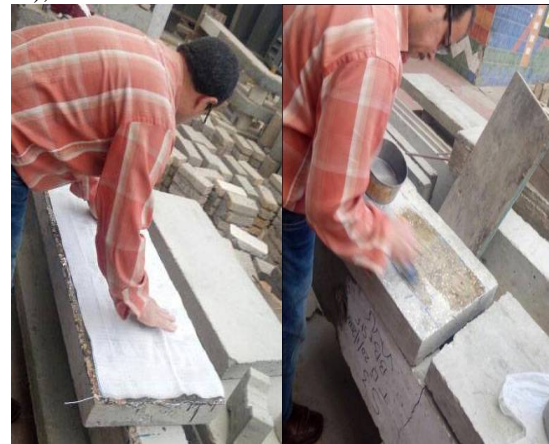
Fig(8):FRP Wrapping around Concrete Elements
