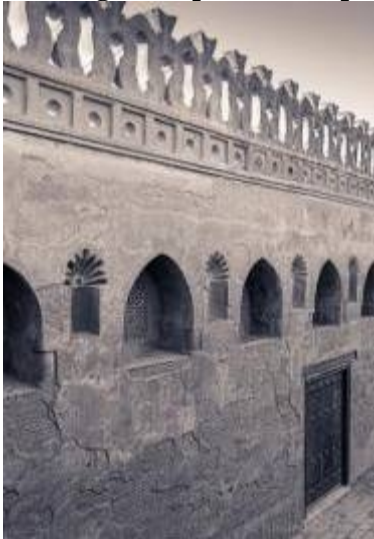
Figure 7: windows of Ibn Tolon mosque
