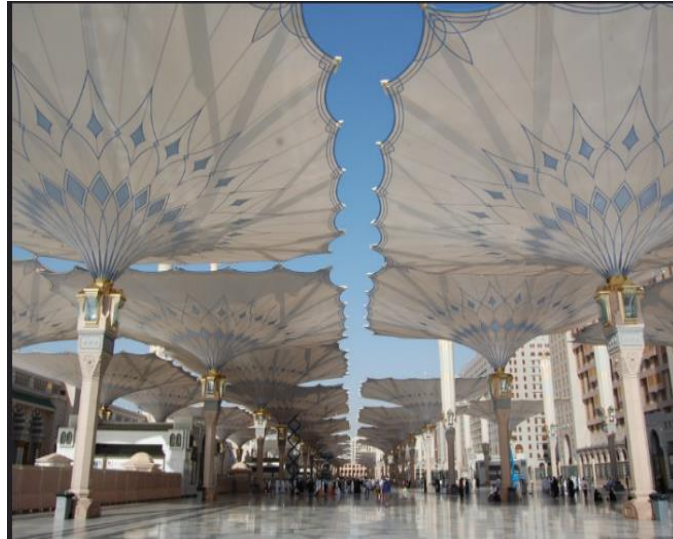
Figure (9) shows the hydraulic umbrellas in the courtyard of the Prophet's Mosque
