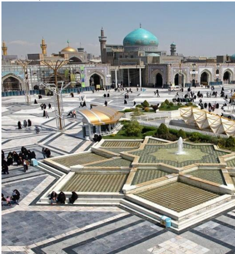
Figure (3) shows the floor design, water feature and seating areas in the courtyard of Imam Reza Shrine, Iran.
