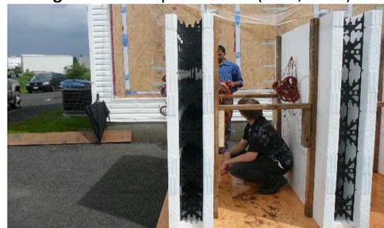
Fig. 8. Insulated Concrete Formwork (ICF) (W. Maref, 2012)
