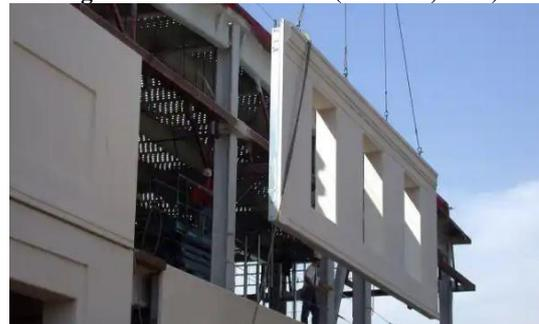
Fig. 4. Prefabricated linear walls (Mishra, 2020)
