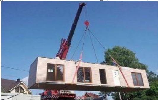
Fig. 2. Single floor Container building (Obinna, 2022)
