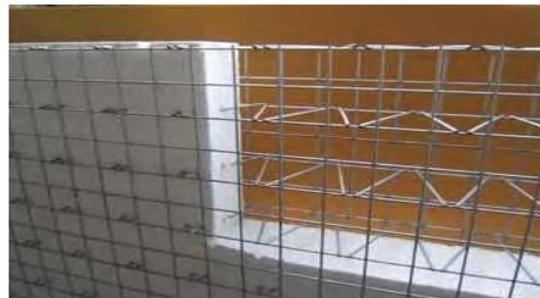
Fig. 7. EPS core panel detail (CBRI, 2017)
