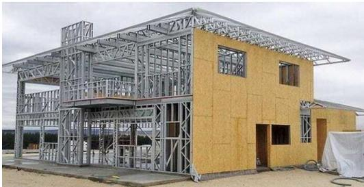
Fig. 5. Lightweight metal structures. (Obinna, 2022)
