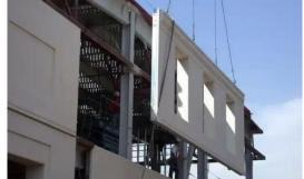
**Fig. 4.** . **Prefabricated linear walls** (Mishra, 2020) 3.2.3. Modular and lightweight structures
