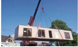
**Fig. 2.** Single floor Container building (Obinna, 2022) 3.2.2. *Prefabricated school buildings*
