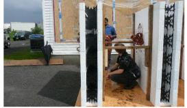
Fig. 8. Insulated Concrete Formwork (ICF) (W. Maref, 2012)
