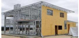
Fig. 5. Lightweight metal structures. (Obinna, 2022)
