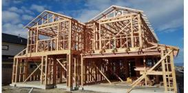
Fig. 6. Lightweight wood structures (Welch, 2022) 3.2.4. Insulated Concrete Formwork (ICF), and Expanded Polystyrene System (EPS)
