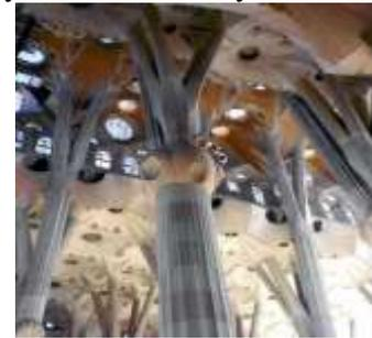
Fig (4) the principles of engineering, which are composed of geometric patterns of straight lines yet produce three-dimensional curved surfaces, were inspired by nature. Antonio Gaudi used these principles to build vaults, walls, and columns.
