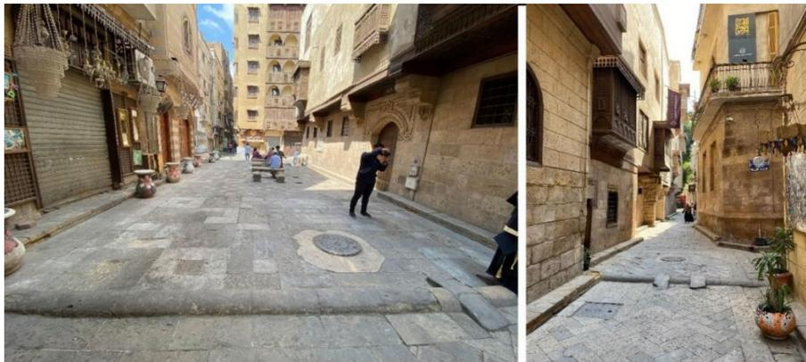
Figures 10 and 11. The stone impervious tiles of Haret Eldarb el asfar, and the location of the manholes.
